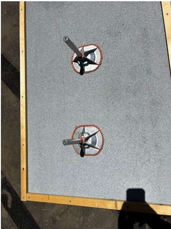
Photo No. 2 Typical OmniShield™ Install w/ Geocel 3500 on Asphalt Roofing
