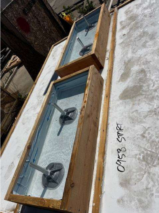
Photo No. 6 Joist/Field Install Submersion Testing of Geocel 3500/ChemLink M1 Installations on TPO
