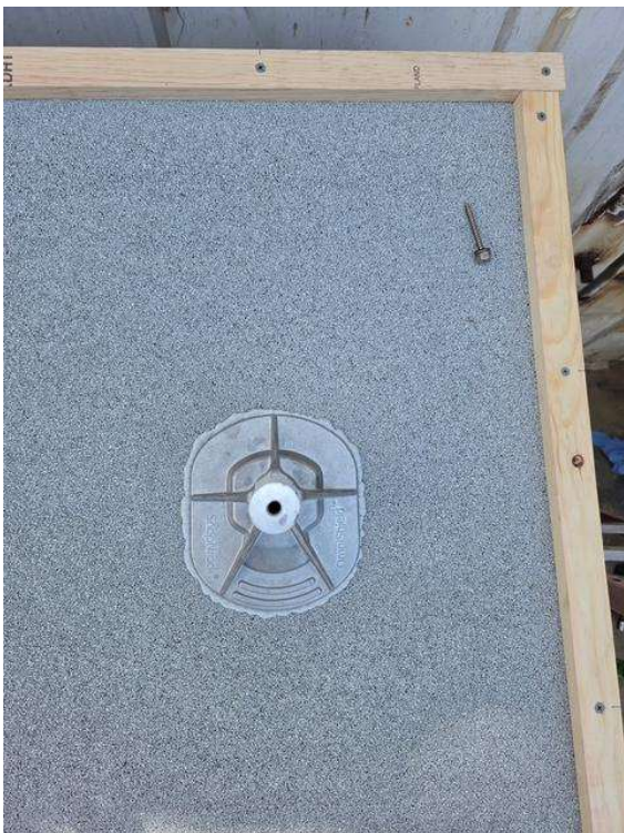
Photo No. 1 Typical OmniShield™ Install w/ ChemLink M1 on Asphalt Roofing
