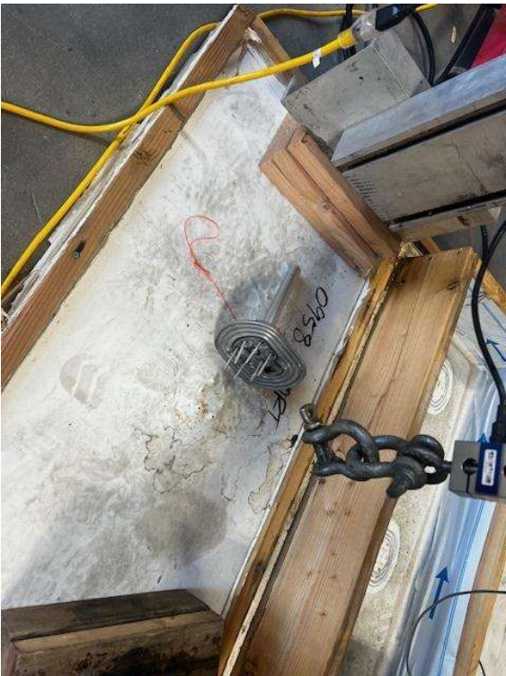
Photo No. 8 Typical Field Condition Failure of OmniShield™ Assembly
